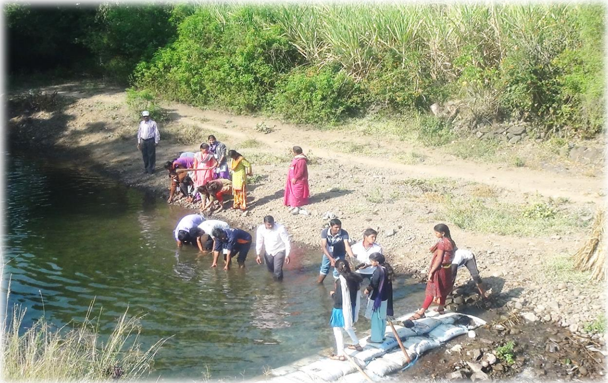
Construction of a Dam on River at the Village of Palshi
